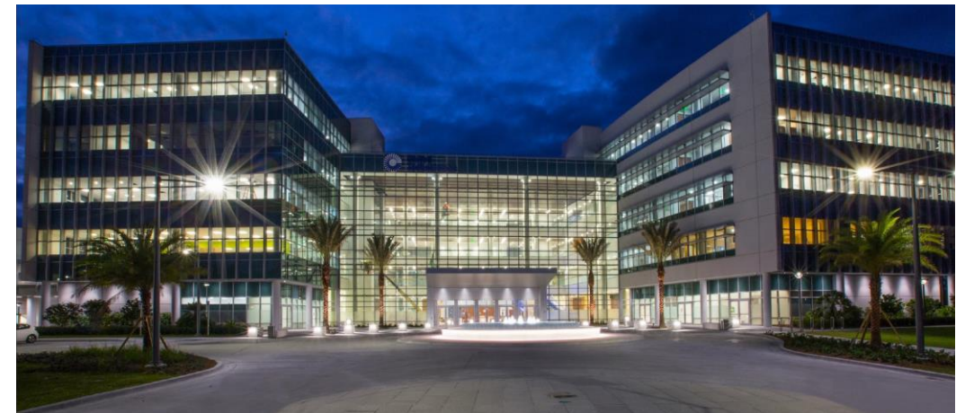
The UTC Center for Intelligent Buildings opened in Palm Beach Gardens, Florida, which serves as the world headquarters for UTC Climate, Controls & Security, and features a broad portfolio of the company's products, as well as a customer experience showcase.
